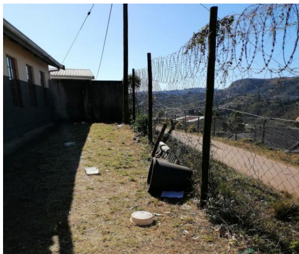
Figure 15: Unused waste bins laying near the fence at school SDO.
