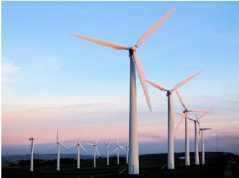
Figure 2: The group of HAWTs in Wind Farm (Sedaghat et al. 2012)
