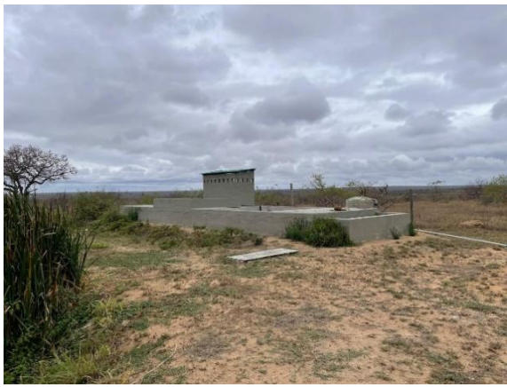
Figure 4.7 Ngala Safari Lodge wastewater treatment plant
