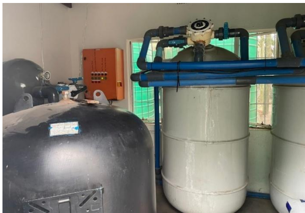
Figure 4.3 Water filtration and pressure system used for lodge water supply Ngala Safari Lodge
