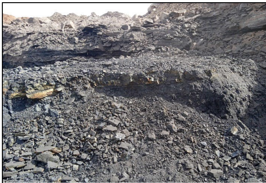
Figure 4.29: Pilot blast of overburden to approximately 0.50 m top of coal
