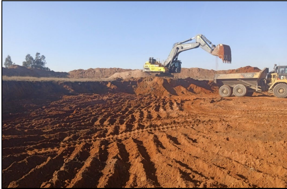
Figure 3.21: Loading time study under soft ground conditions at Mine 1
