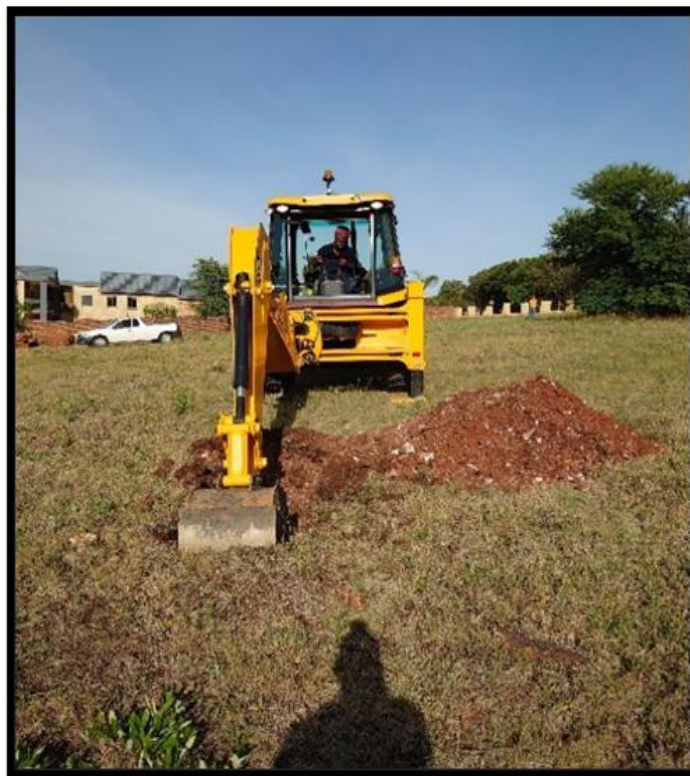
Figure 3.5: Excavation of the test pit
