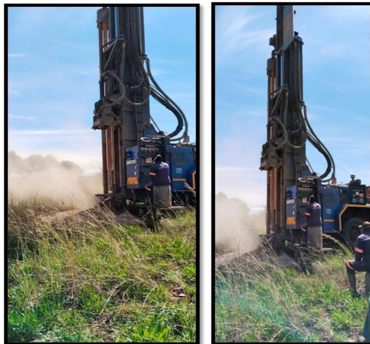
Figure 3.8: Rotary-percussion drilling
