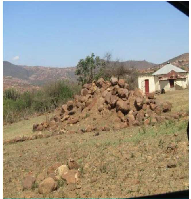
Photo 4.4 Boulders emanating from construction activity are stockpiled for reuse within the household
