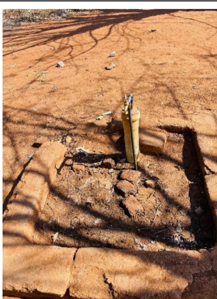
Image 8: Poor infrastructures (Non-functional water tap)
