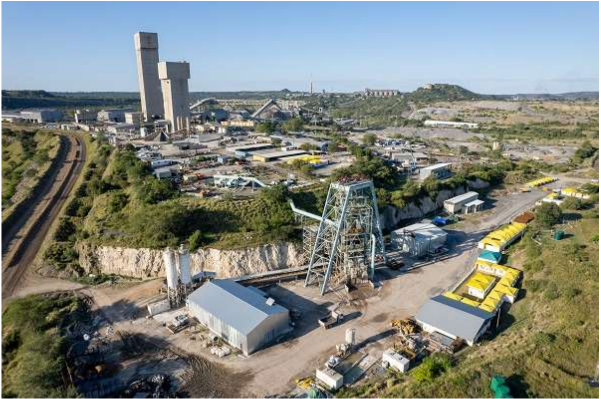
Figure 1.1 – Aerial view of the PMC Ventilation Shaft with Service and Production Shafts in the background (Source: PMC, 2024)
