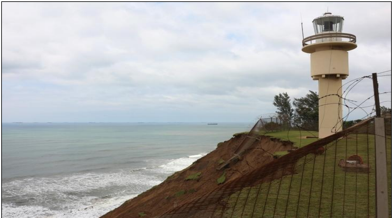
Figure 3.15: The Richards Bay Lighthouse was demolished due to its imminent collapse. Built in 1979, standing 200 m from the edge of the cliff, it was demolished in 2018, standing a mere 5m from the sea cliff edge (Zululand Observer Newspaper, 2017).
