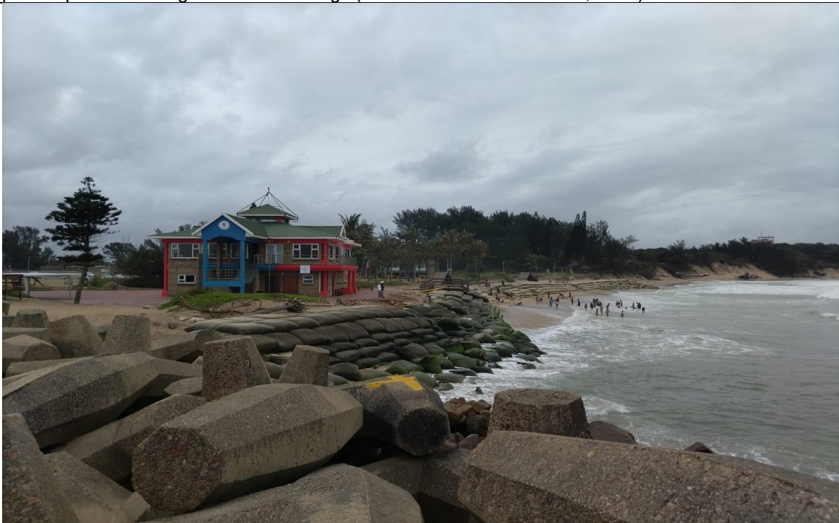
B: Geotextile sand bag placement in 2015 creating an artificial slope (Source: Alakram, 2023).
