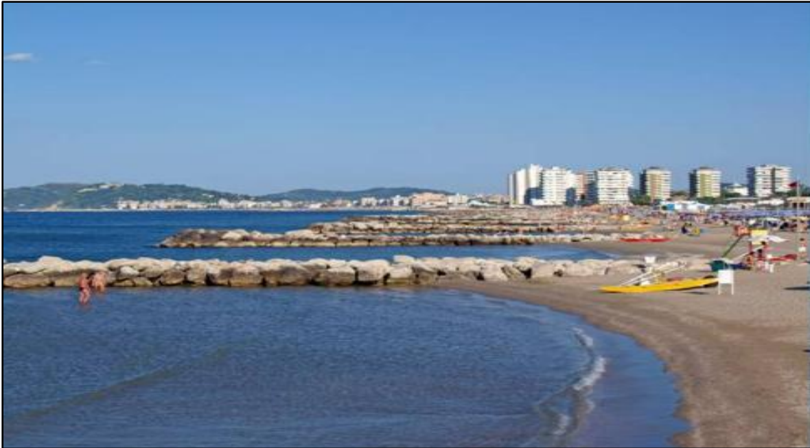
Figure 5.15: A series of breakwaters in Croatia (Pranzini & Margeta, 2022).
