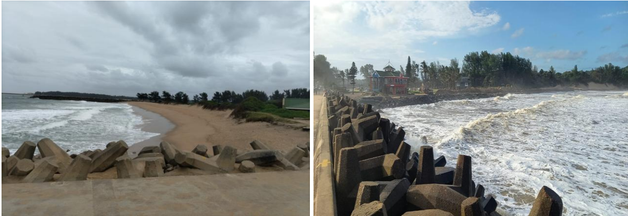
Figure 3.10: Dolos breakwaters in Richards Bay (Alakram, 2024).
