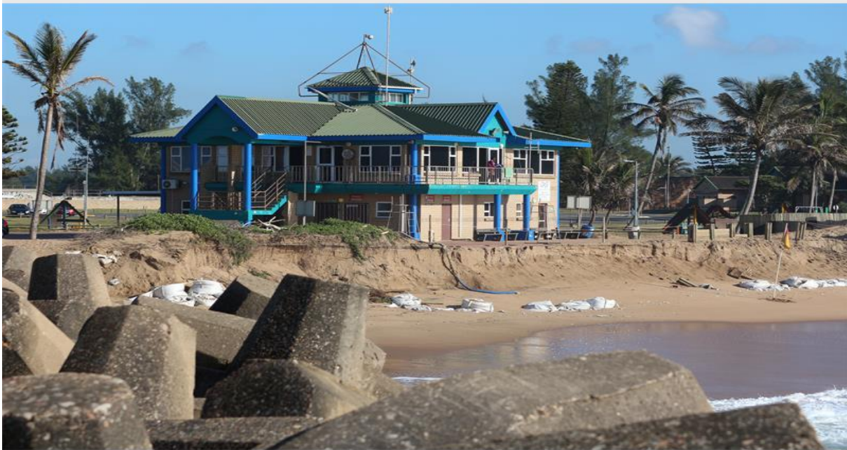
A: 2015: Lifeguard tower in Alkantstrand North beach facing immediate threat from coastal erosion and prior to placement of geotextile sand bags (Source: Zululand Observer, 2015).
