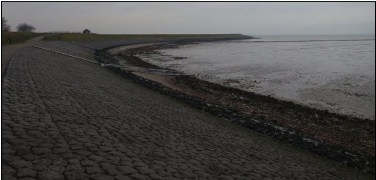
Figure 2.2: Armoured sea dikes in the Netherlands at low tide (Hanegan, 2010).
