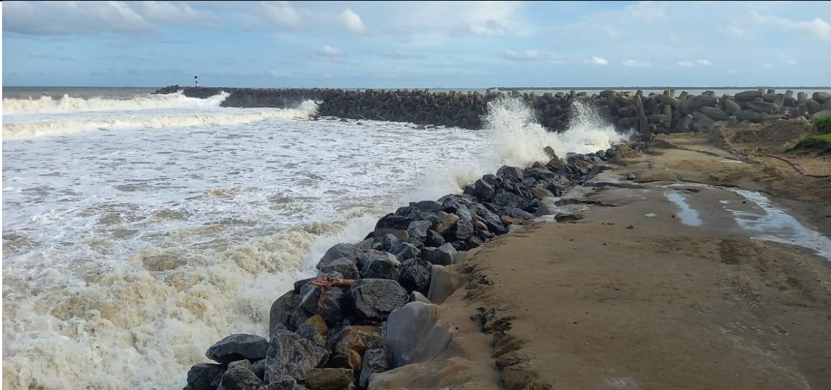
D: 2025 - A combination of geotextile sand bags and rock revetments as a recent strategy. Sand replenishment was undertaken landward of the rocks. (Alakram, 2025).
