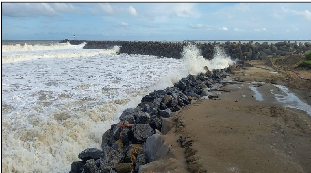
Figure 5.13: Rock revetments as a coastal protection strategy in Richards Bay (Alakram, 2024).
