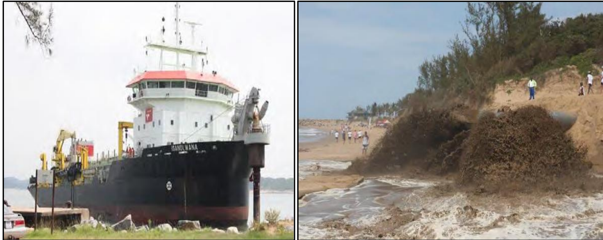
Figure 5.12: Left: The hopper dredger docked inside the harbour and connected to the discharge pipeline. Right: Sand is pumped onto Alkanstrand beach via the discharge pipeline. Adapted from Wells (2015).
