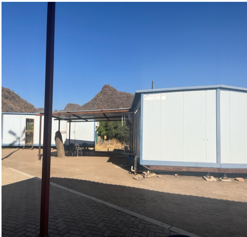
Figure 19: Ga-Seroka Clinic infrastructure
